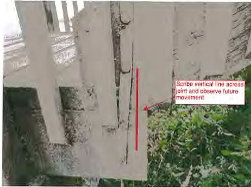
Figure 1 – Scribe Line for Movement Indicator
