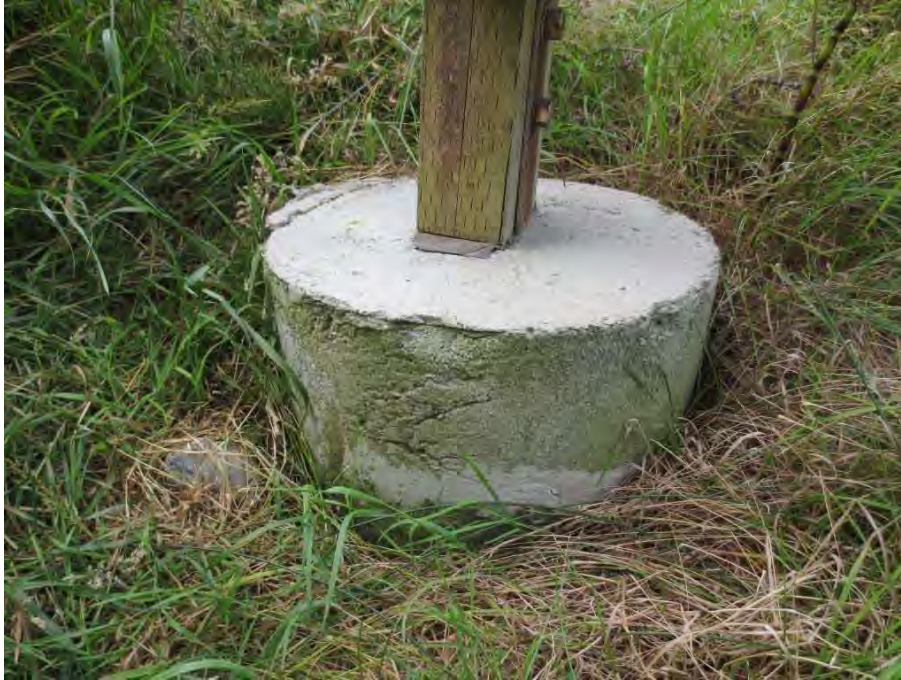
Photo 9 – Typical Concrete Footing
