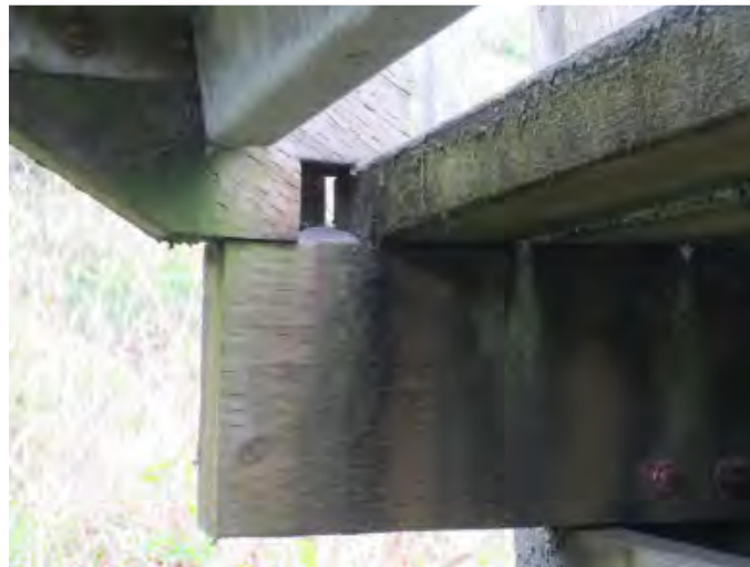
Figure 5 – Typical Bearing Seat Connection
