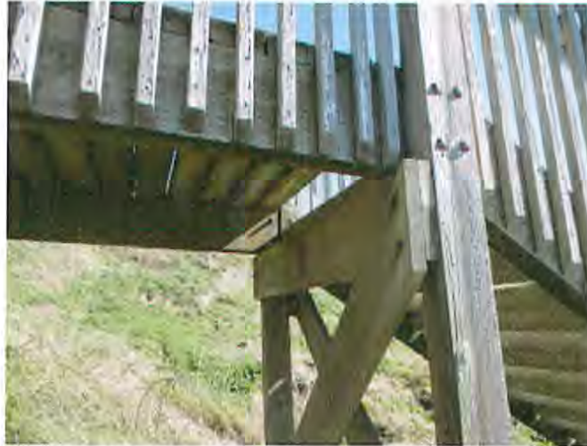
Figure 4 – Typical Bearing Seat Connection
