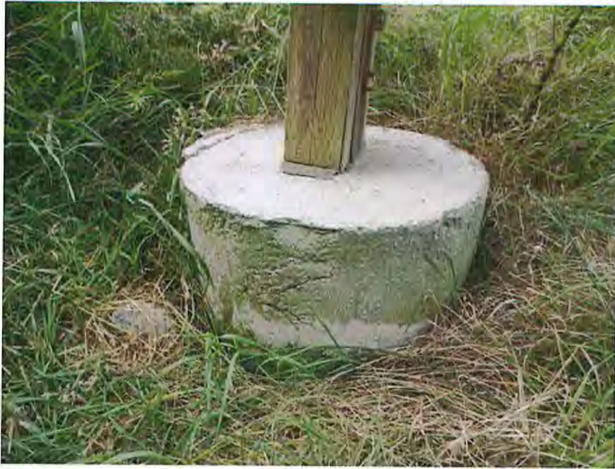
Photo 9 – Typical Concrete Footing
