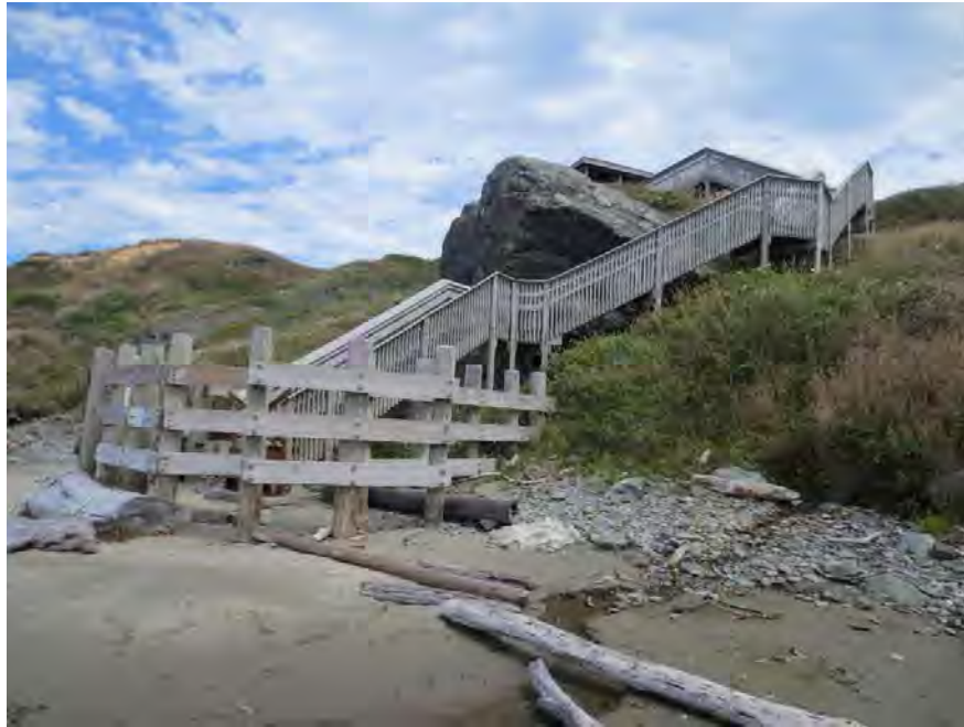
Photo 1 - View from Base of Structure
