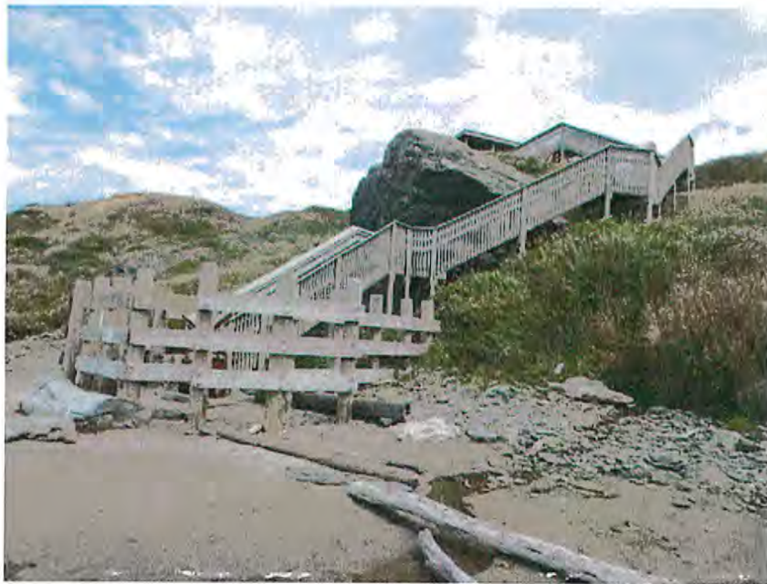
Photo 1 - View from Base of Structure
