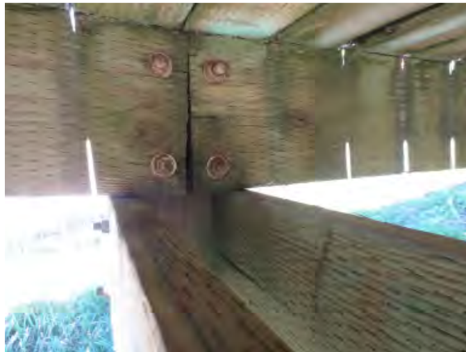
Figure 3 – Typical Bearing Seat Connection
