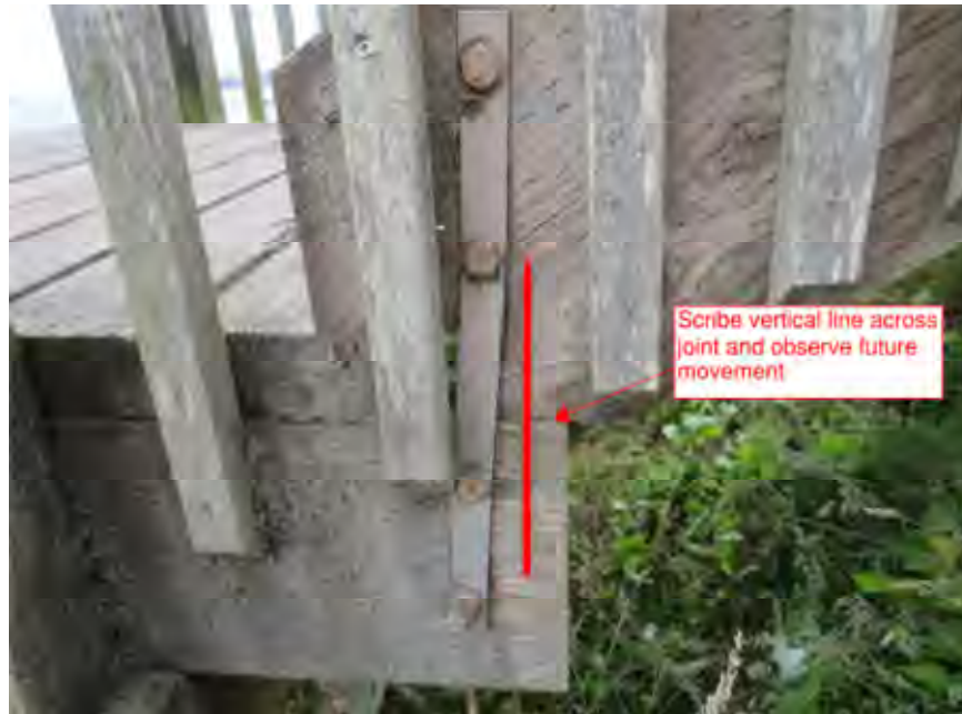
Figure 1 – Scribe Line for Movement Indicator
