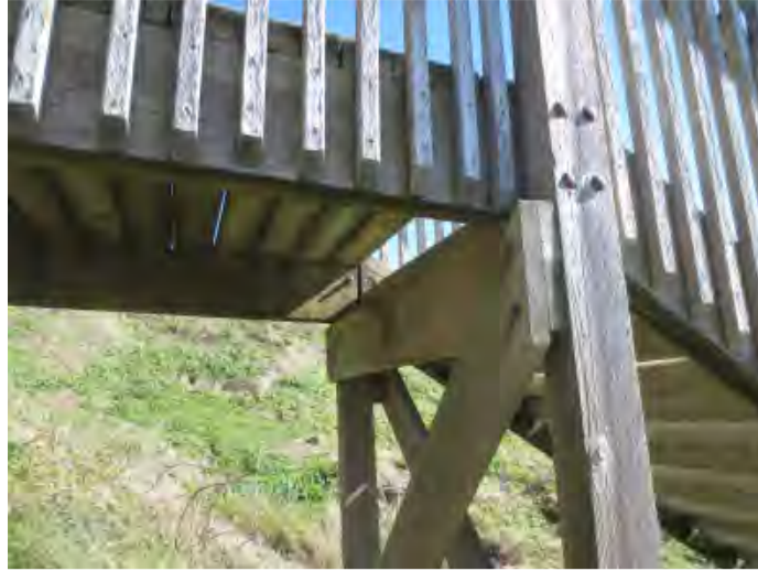
Figure 4 – Typical Bearing Seat Connection
