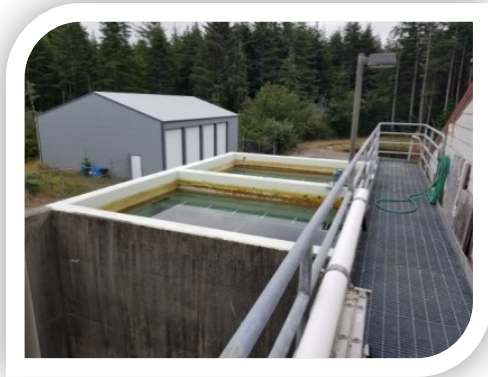
FIGURE 5.3.4 DUAL MEDIA FILTERS
