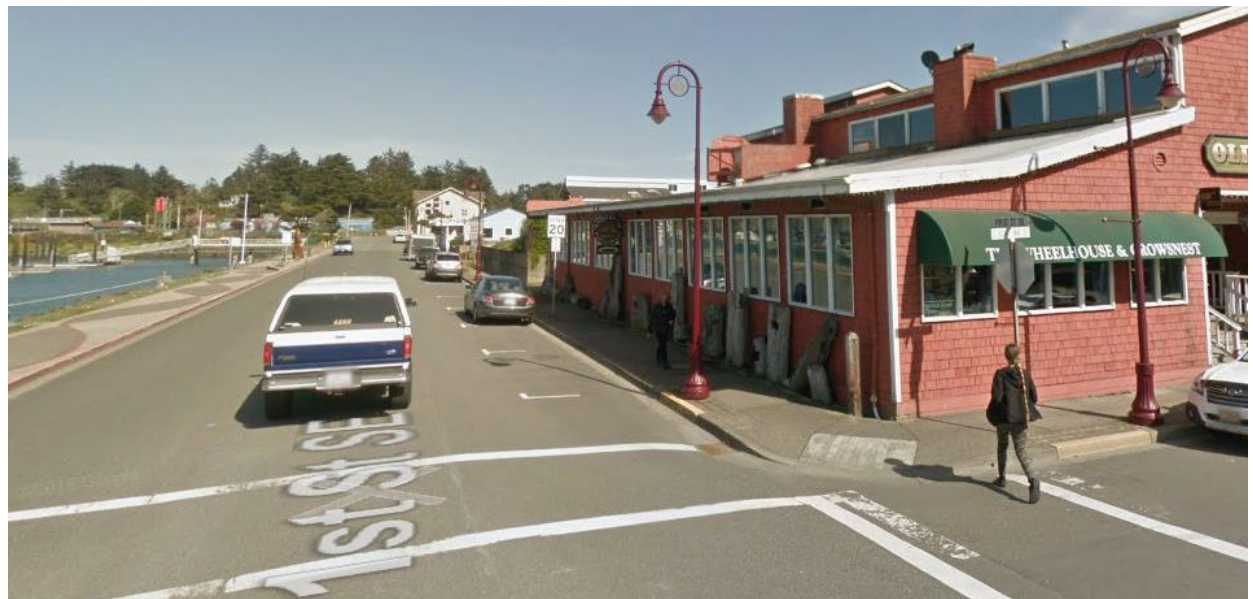
Figure 3-15. Pedestrian-Scale Lighting in Old Town Bandon
