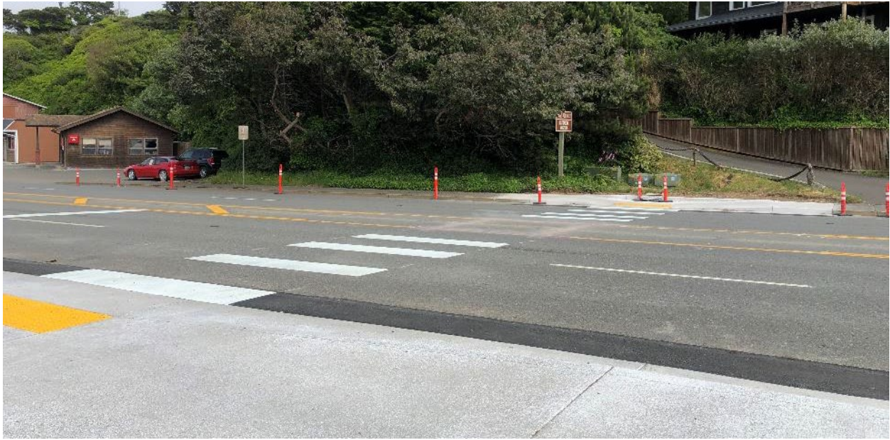
Figure 3-14. U.S. 101 Crossing Near Chicago Avenue
