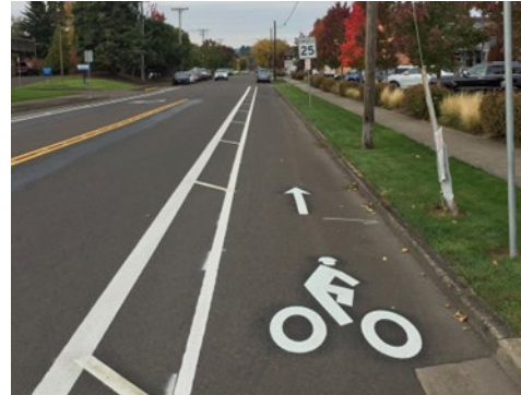
Photograph 4-1. Buffered Bike Lane
