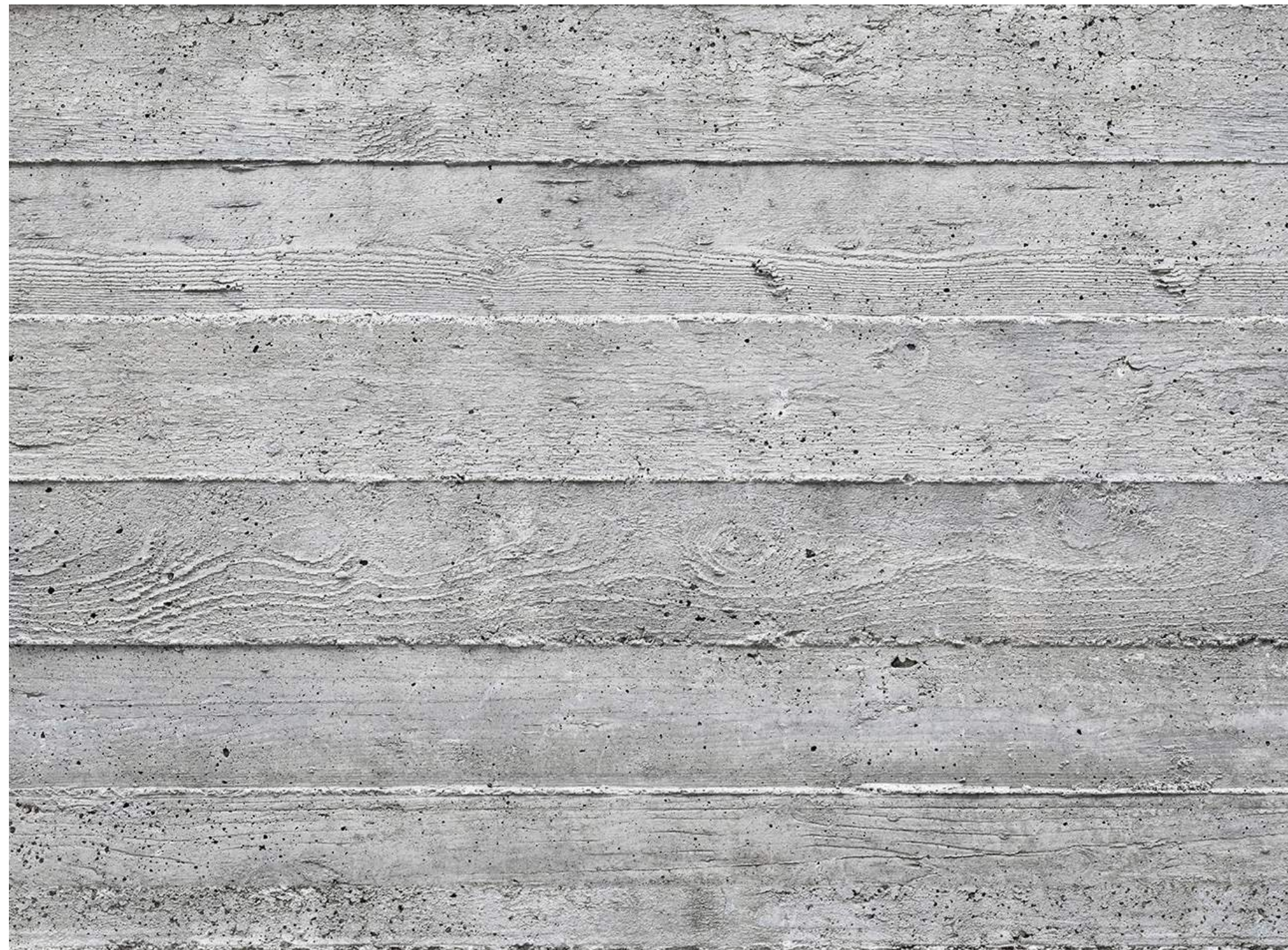
BOARD FORM CONCRETE
