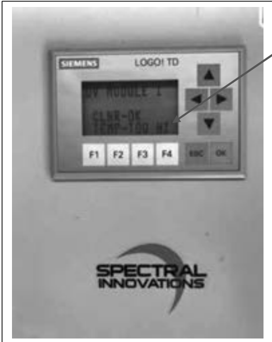
Critical UV system data is local to the control panels. No output alarm signal to SCADA or Auto Dialer.
