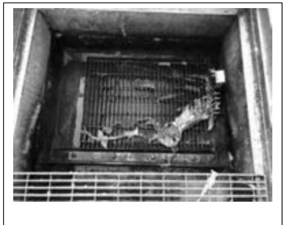
Manual Screen with no flow
