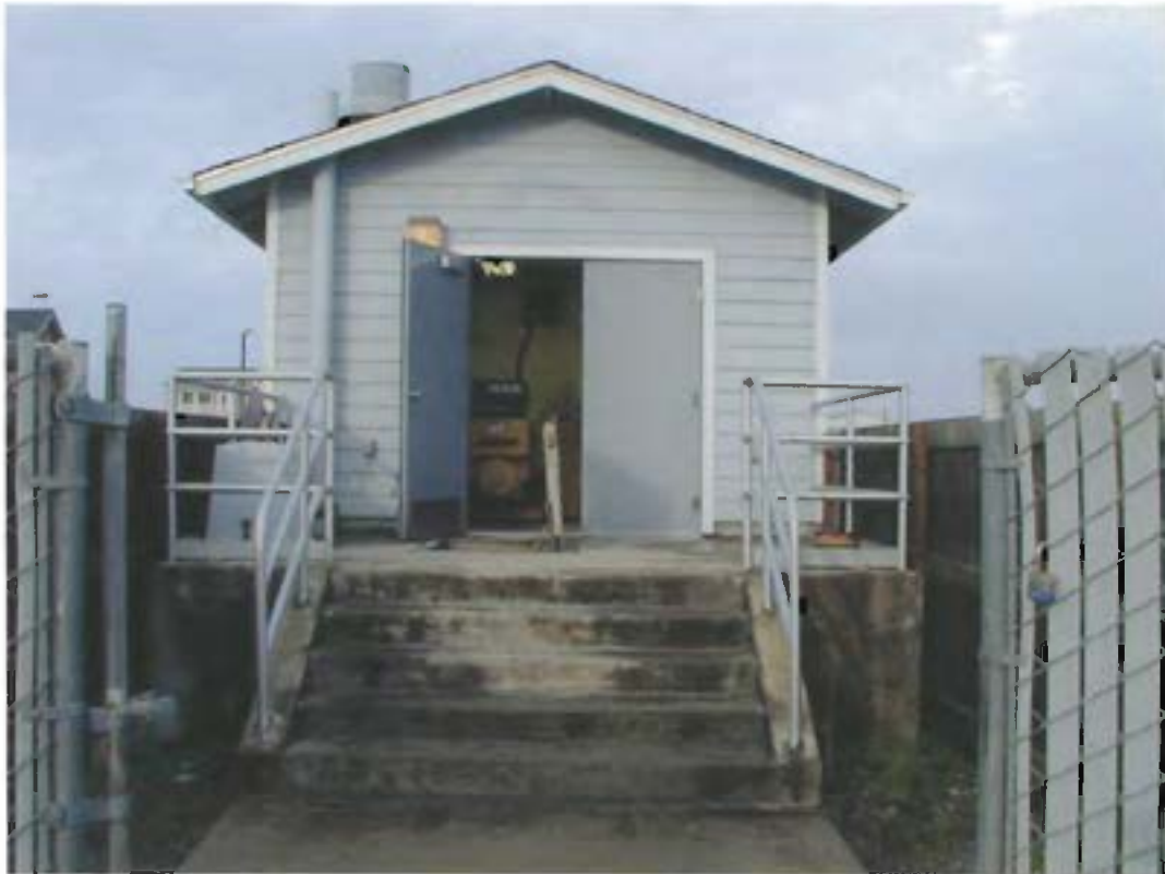
South Jetty Pump Station
