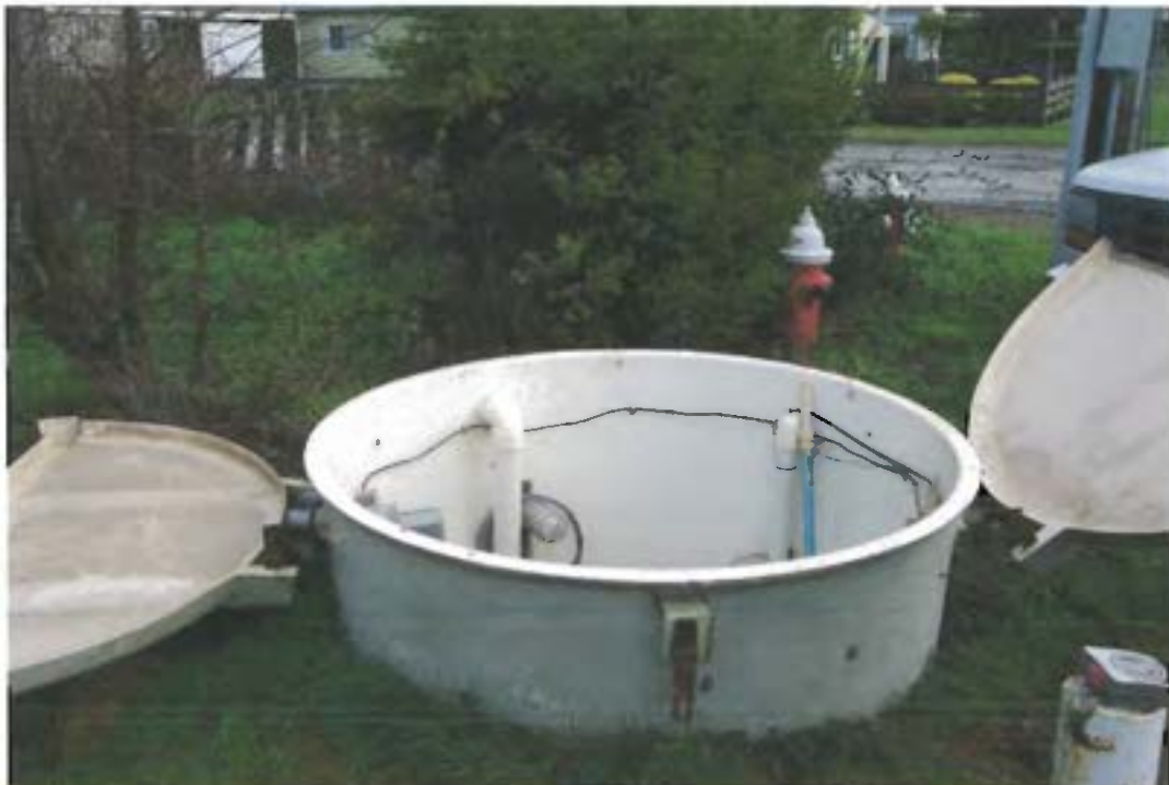
North Street Pump Station
