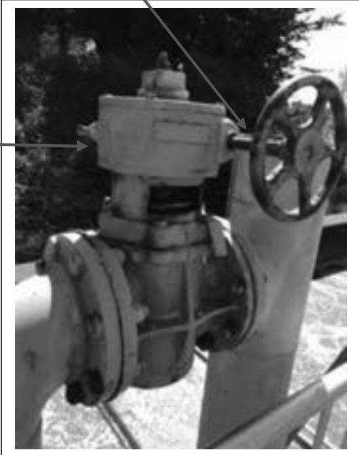
Moderate to severe corrosion occurring to mud valve stems.
