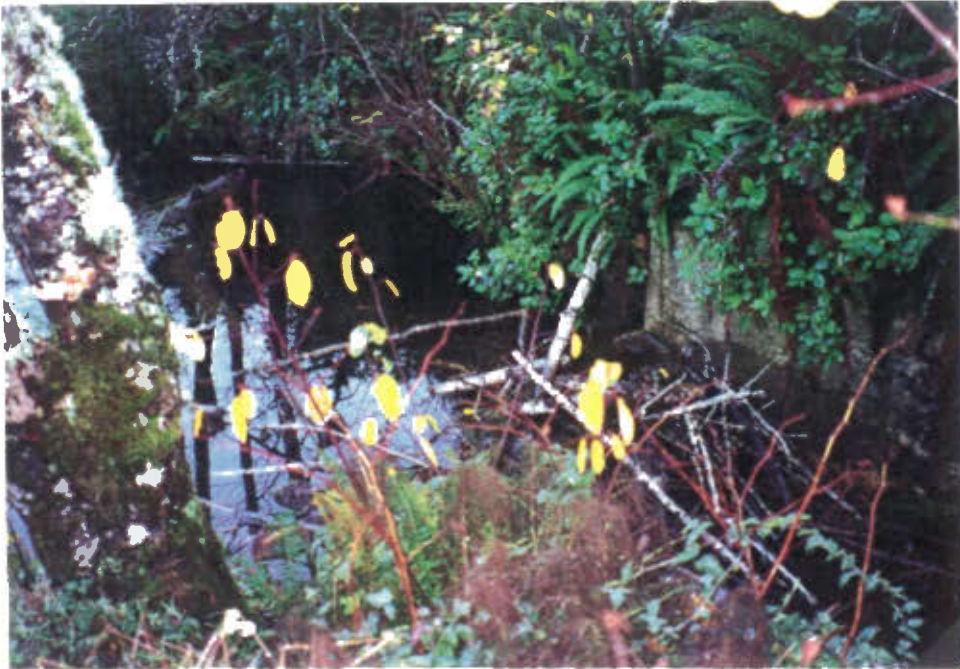
PHOTO 7-5. FERRY CREEK DAM SPILLWAY
