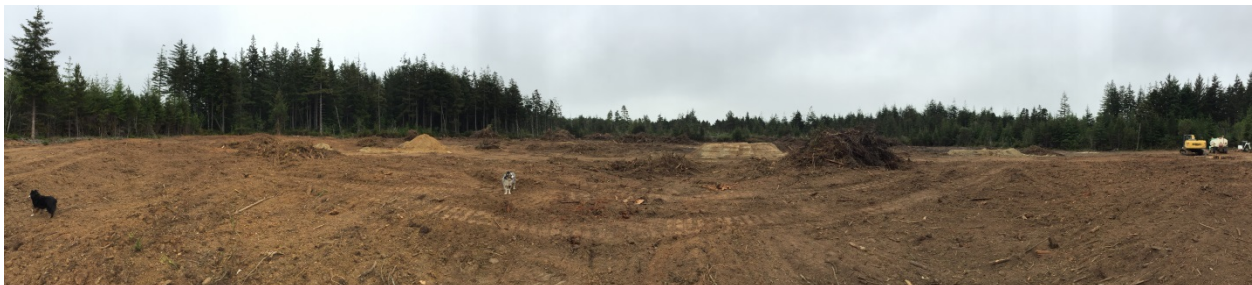
Panoramic view of Lot 2400 after brush was cleared in May 2014.
