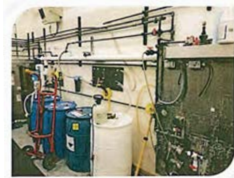
FIGURE 5.3.2 POLYMERS ADDITION
