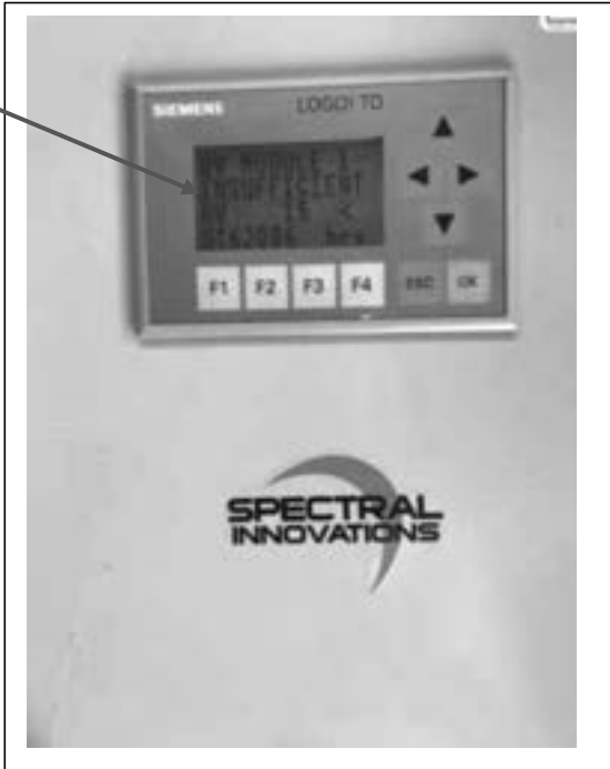
Critical UV system data is local to the control panels. No output alarm signal to SCADA or Auto Dialer.
