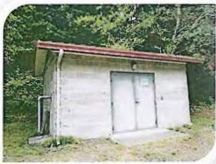
FIGURE 5.2.2 LOWER PUMP STATION
