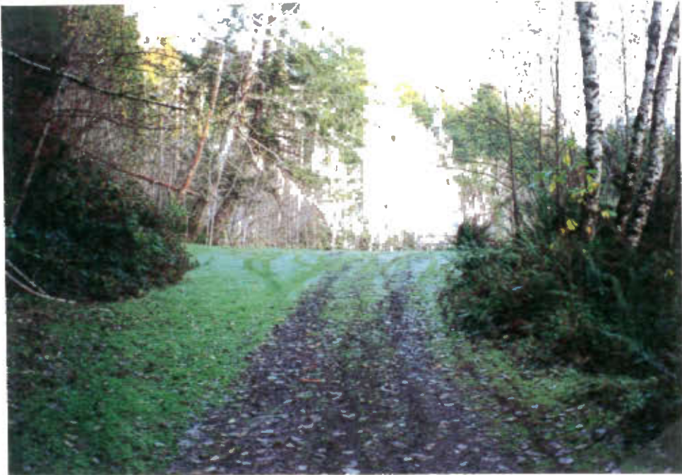
PHOTO 7-1. FERRY CREEK DAM
