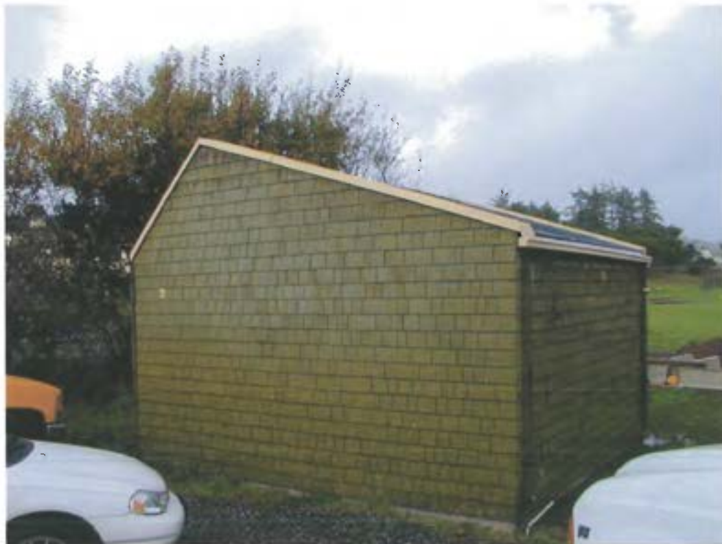
Johnson Creek Pump Station
