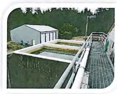
FIGURE 5.3.4 DUAL MEDIA FILTERS
