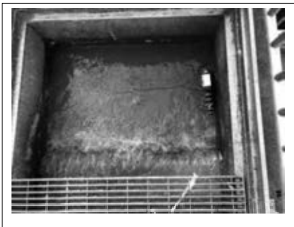
Manual Screen with flow
