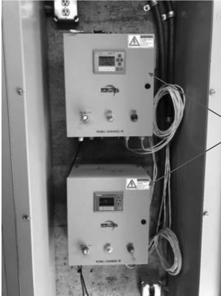
Critical UV system data is local to the control panels. No output alarm signal to SCADA or Auto Dialer.
