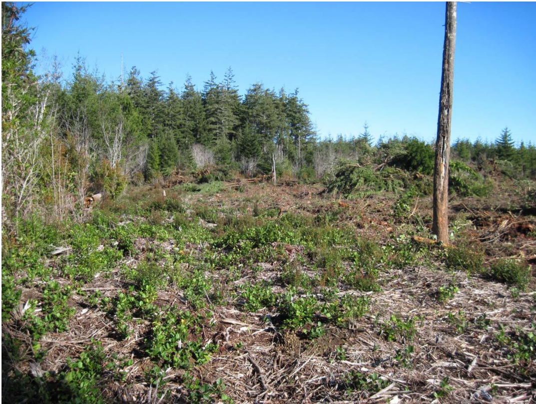
Photo 3. View of site after brush clearing
