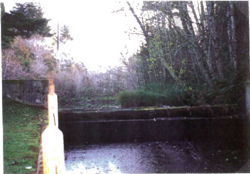
PHOTO 7-6. GEIGER CREEK DAM SPILLWAY
