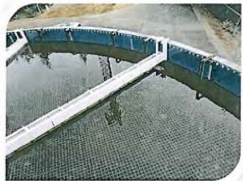
FIGURE 5.3.3 CLARIFIER EQUIPMENT
