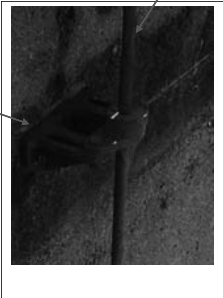
Moderate to severe corrosion occurring to mud valve stems.
