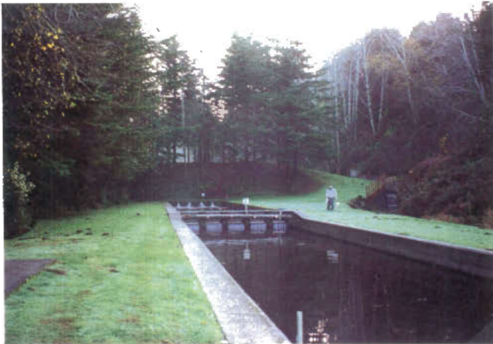
PHOTO 7-3. GEIGER CREEK DAM
