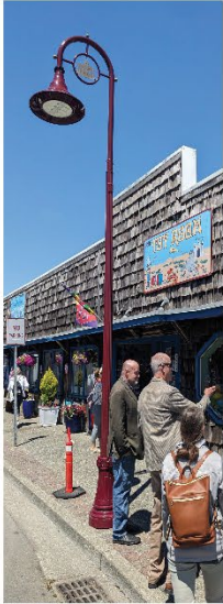
EXISTING STREET LIGHT
