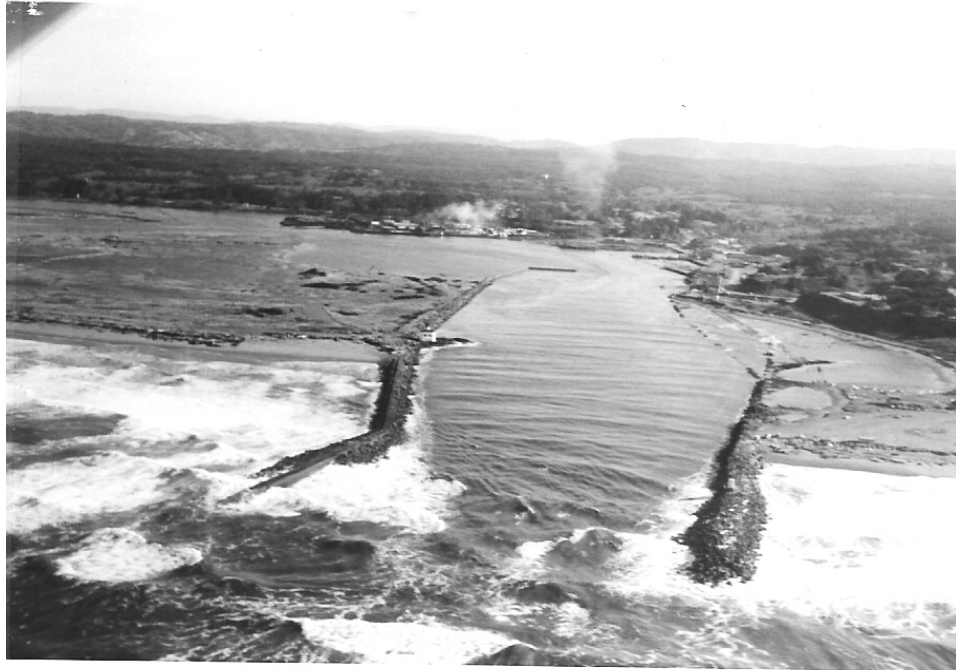
The jetties and harbor entrance, showing strong cross currents at the bar.
