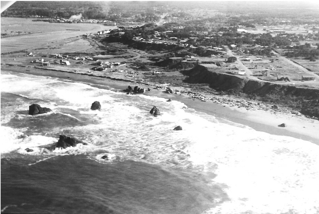
Breakwater Addition (South Jetty) and the Bluff.
