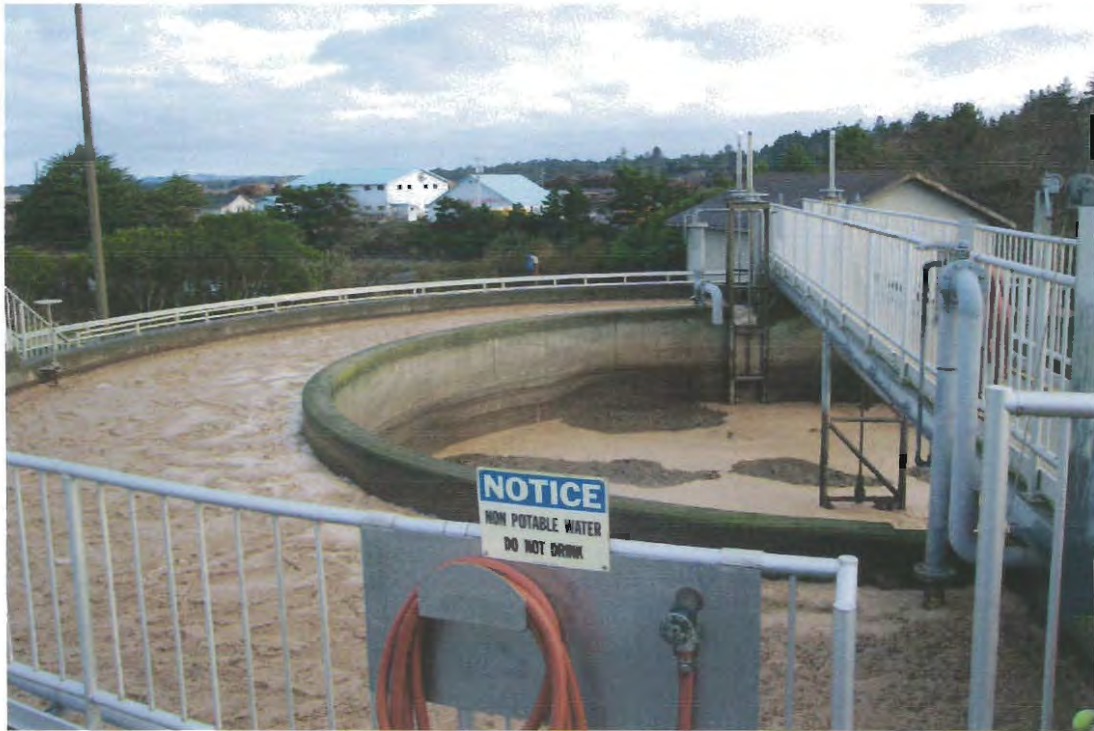
Bandon WWTP Digester
