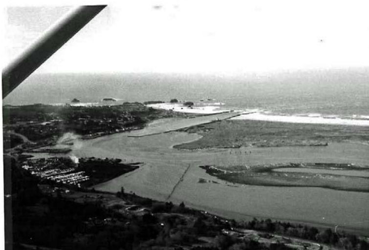
Coquille River estuary. Moore Mill at left/Oregon ocean island rocks offshore. Estuary tideflats flood lands in foreground.
