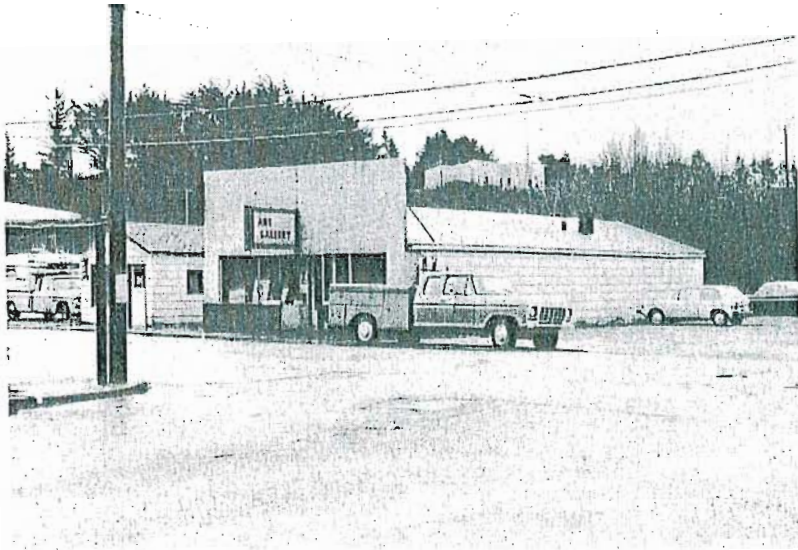
Existing Structure on 2nd Street
