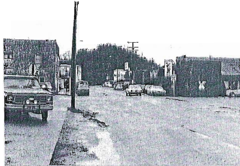
Looking West on 2nd Street
