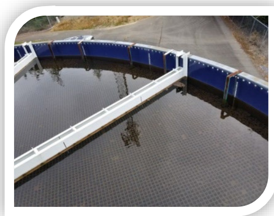
FIGURE 5.3.3 CLARIFIER EQUIPMENT
